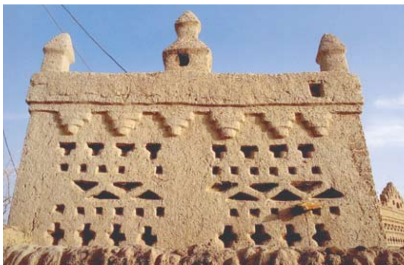
The window and light holes of a two storey building, Saravan
